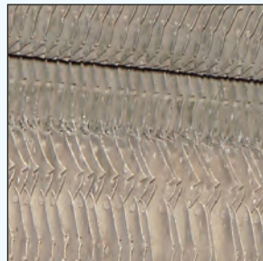
The visible foam, clean and evenly distributed, allows the Finfoam technician to confirm a "top quality" job.
